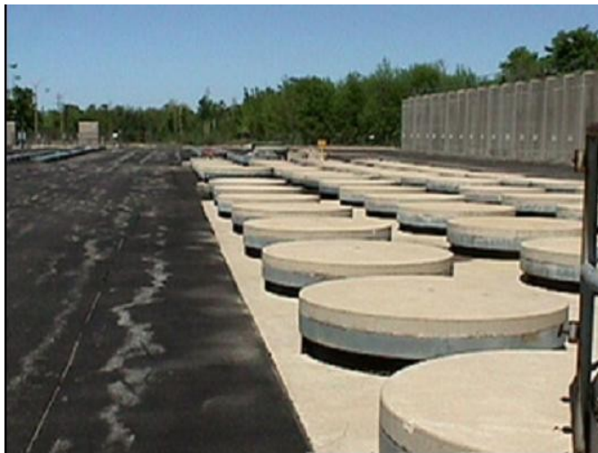
Figure 3.1-3: In-ground Containers for Intermediate-level Waste Storage
