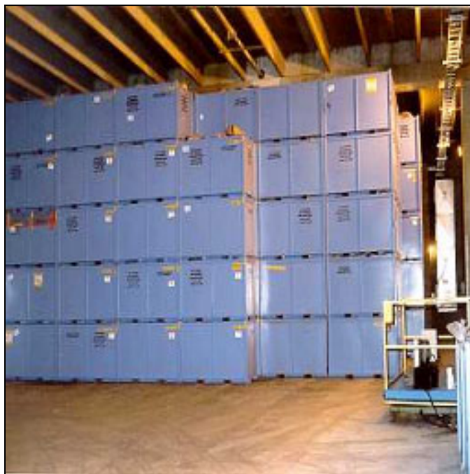
Figure 3.1-2: Containers Stacked Inside Low-level Storage Building
